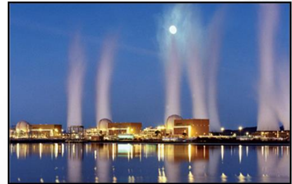
Palo Verde Nuclear Generation Station
